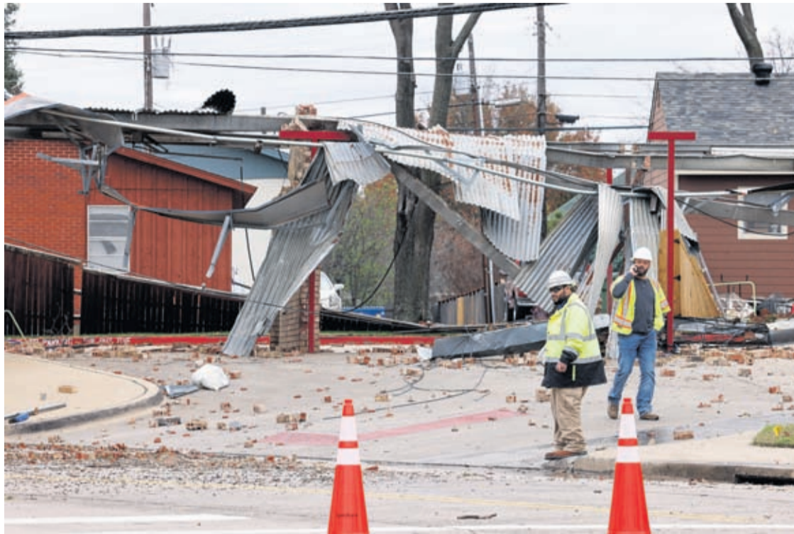
Crews survey damage from a possible tornado in Grapevine, Texas, Tuesday, Dec. 13, 2022.
